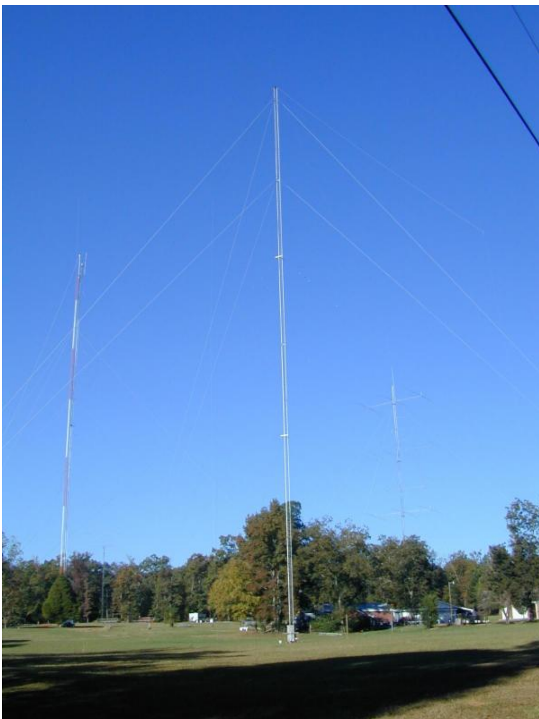
From Left to Right: 300' Tower, 220' 160m Vertical and 200' Rotating Tower
